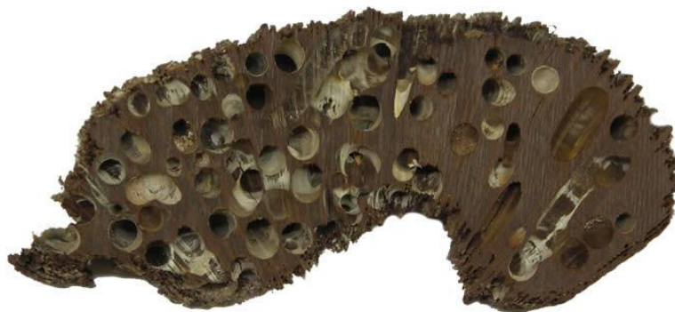
Marine borer damage to a hardwood pylon
