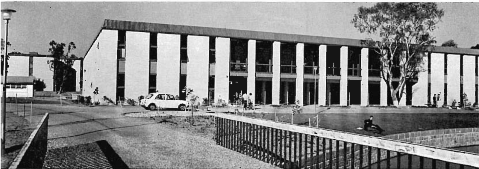
Above: The Union Building at La Trobe University. Cedar windows were protected during construction by plywood panels. Concrete formwork was plastic faced plywood.
