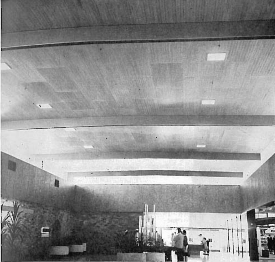
Left: Perforated plywood acoustic ceiling in the "Gallery" section of Northland shopping centre.
