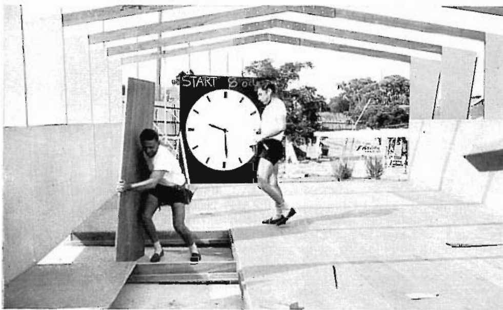
One and a half hours after building begins, the foundation and frame are complete, and plywood in-fill panels are installed.
